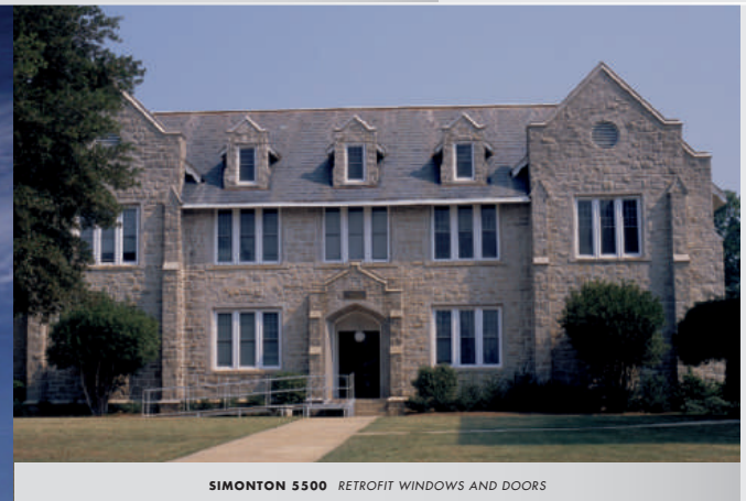
SIMONTON 5500 RETROFIT WINDOWS AND DOORS
